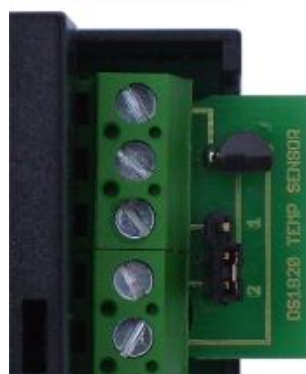
Detail of installation
